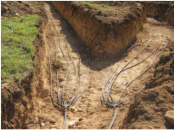
Installing a horizontal loop GSHP can be cheaper than the extensive drilling required for a vertical loop field, but it does require more land. Image courtesy Geoexchange
